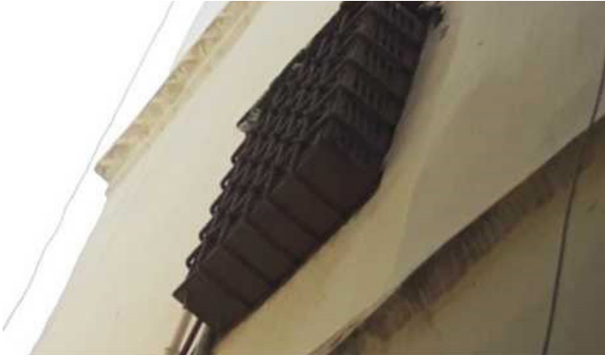
A window of a house in Al Casbah dating back to the Ottoman period
