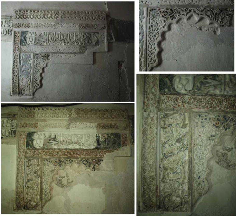
Figure 5: Blind mihrab in the qiblah wall east of the minbar; upper left- general view of the plaster before cleaning; lower left- general view of the plaster after cleaning; upper right- detail view of the multifoil arch before cleaning; lower right- detailed view of the frame with interlaced carnations and tulips after cleaning.
